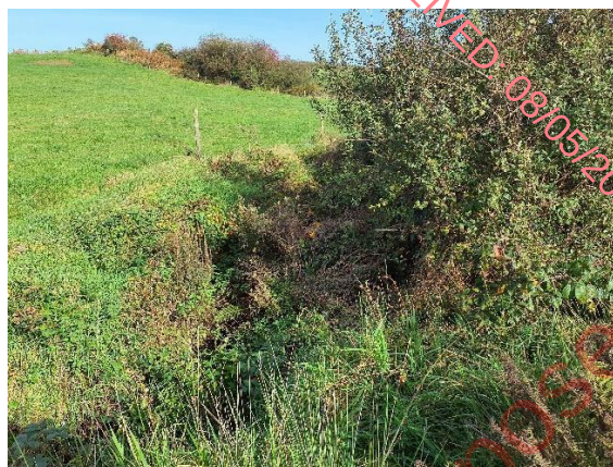
Plate 2. Site 1 inaccessible section, downstream of road crossing
